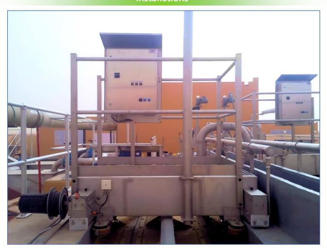
The grit and grease removal bridge Omega GGRB from EMO is designed to be used in grit and grease removal installations from municipal and industrial wastewater treatment plants.
